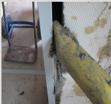
Filling of frame joints
