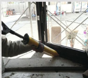
Filling of frame joints
