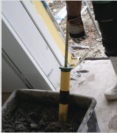
Filling the gun with mortar
